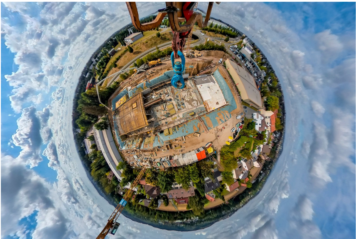
Photos of the construction progress: BORA / Sascha Schürmann
